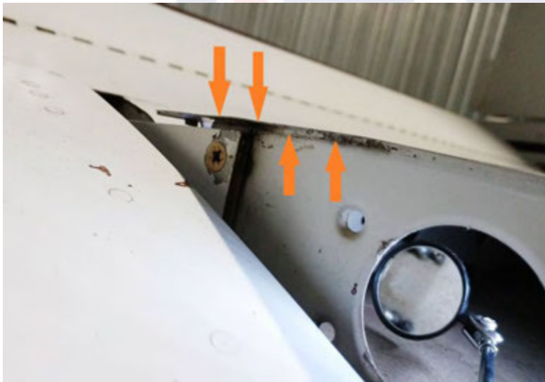
Photo: Check for delamination.jpg
